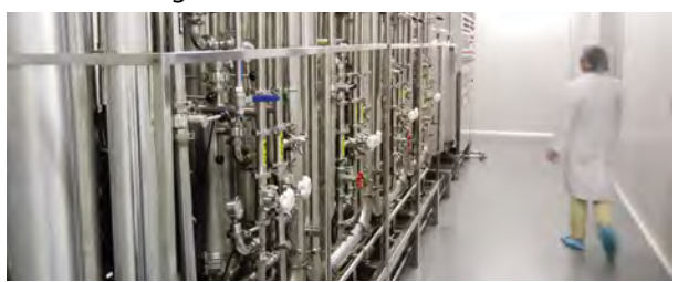
FITT control room and extraction tanks
